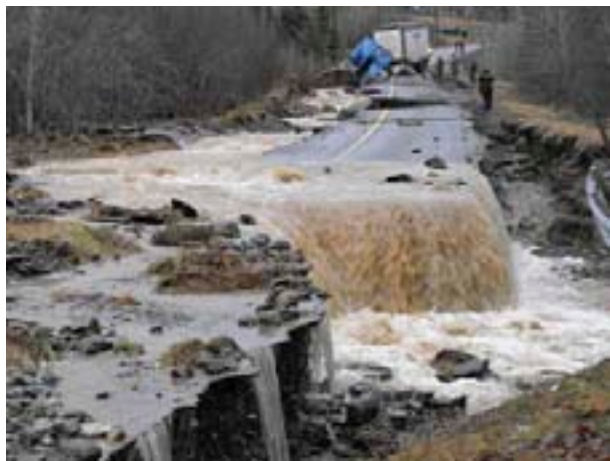
High water levels from extreme rainfall event washed out a road in Northampton, December 13–14, 2010.
