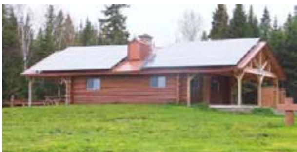
Solar panels installed at Mount Carleton Provincial Park.
