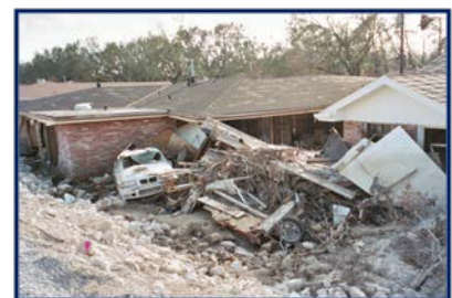
Canal levee breaches as a result of Hurricane Katrina in New Orleans in 2005. Note damages can be more extensive due to high velocity flood flows than if the levee was not there.
